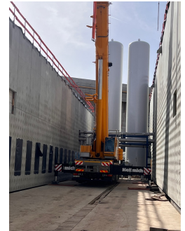
6 He tanks of the cryo facility were installed, Apr'24
