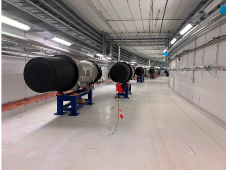
installation of SIS100 dipoles Apr'24
