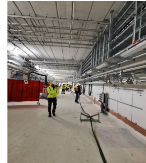
start of cable pulling work, Q3/23
