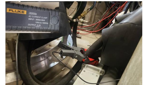
AC current clamp installed at VMTF
