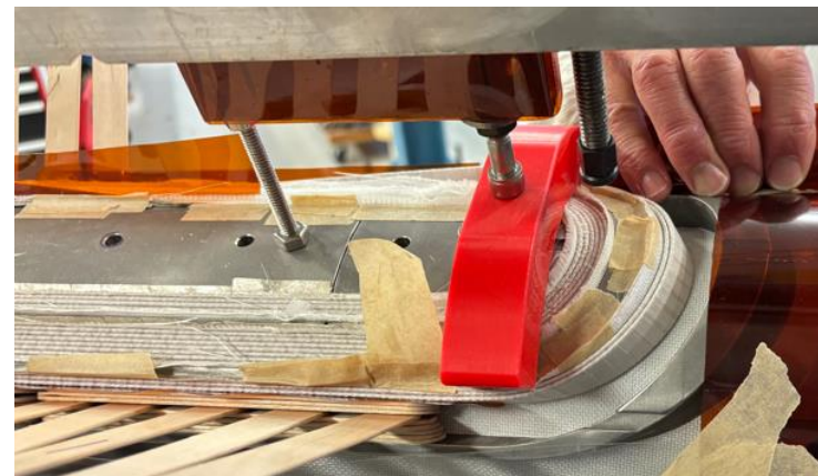
Cable winding around return end area
