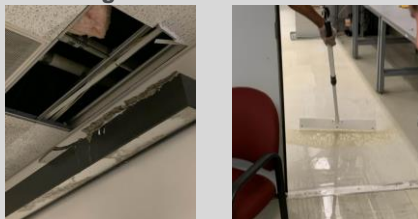
Water Damage to Ceiling Tiles and Pooling in Labs on Floors Below
