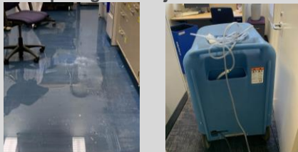
Water Damage to Ceiling Tiles and Pooling in Labs on Floors Below
