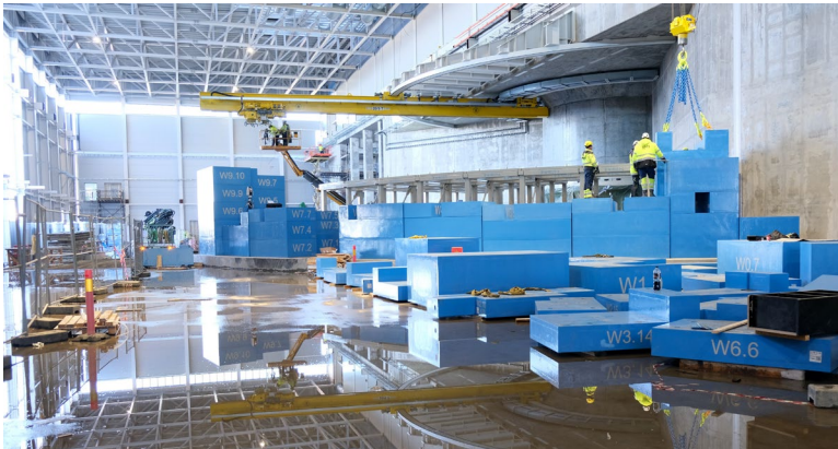
Installing bunker shielding blocks at ESS
