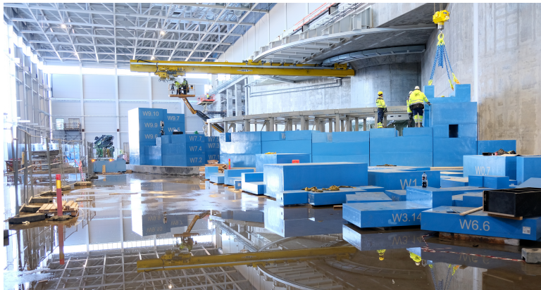
Installing bunker shielding blocks at ESS
