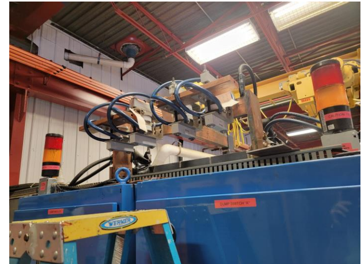
Bus bar at the PS, design and preparations for installing a by-pass line
