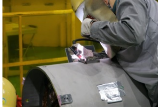
Welding of alignment markers
