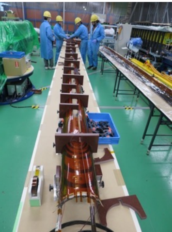
QPH, ground insulation wrapping
