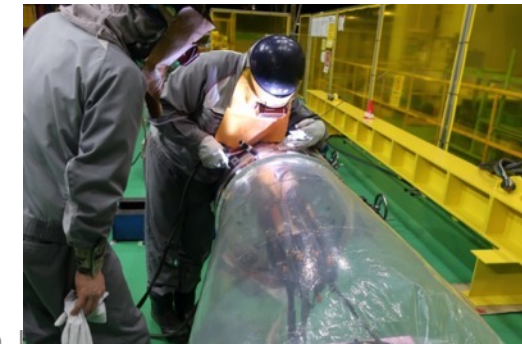
End ring welding
